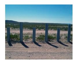
"bollard" style made up of closely spaced, large-diameter vertical posts. Our nearly 2,000 mile long southwest border (696 miles land and 1295 miles of river) is now secured by 354 miles of primary pedestrian fencing, 82 percent (290 miles) of bollard design, and by 300 miles of primary vehicle fencing (225 miles of a more impervious, modern design.)
